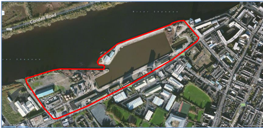
Figure 3 Aerial view of Limerick Port
